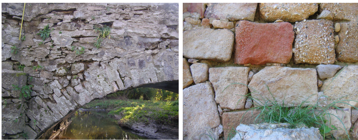
Fig. 2. Damages: cracked spandrel wall (left), Mortal loss on (right)
