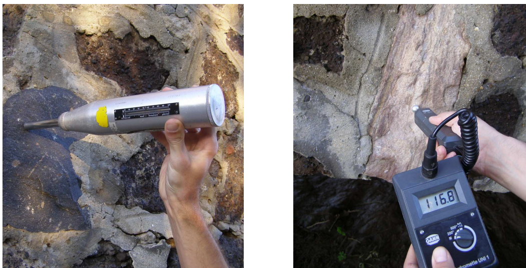
Fig. 1. Schmidt hammer test (left), Moisture content measuring (right)
